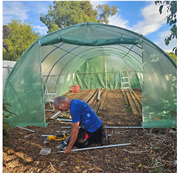
Rob working on the new tunnel house
